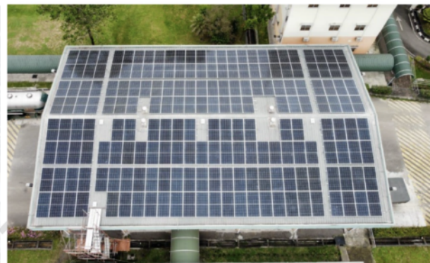
Solar Modules Installed at Weight Bridge Roof.
